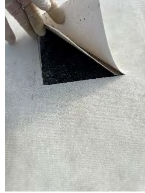
Upper East Roof
