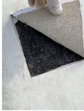
Upper East Roof
